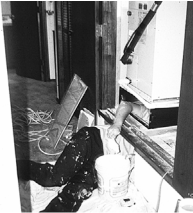
Lining a panned cavity: Foil-faced foam board designed for lining duct cavities is sealed with duct mastic to provide an airtight, insulated return.
