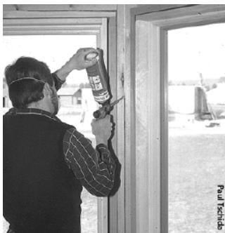
One-Part Foam: A contractor uses an applicator gun to seal spaces between framing members and around windows.
